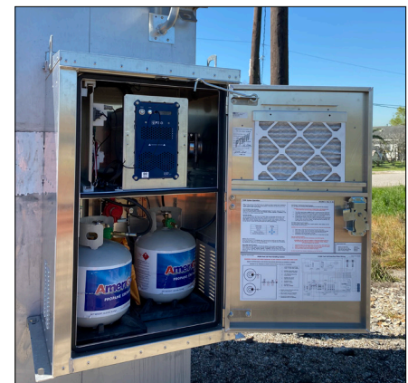
The P250i Solid Oxide Fuel Cell is housed inside of an NEMA outdoor rated enclosure that can be foundation, pad or bungalow mounted (pictured above).
