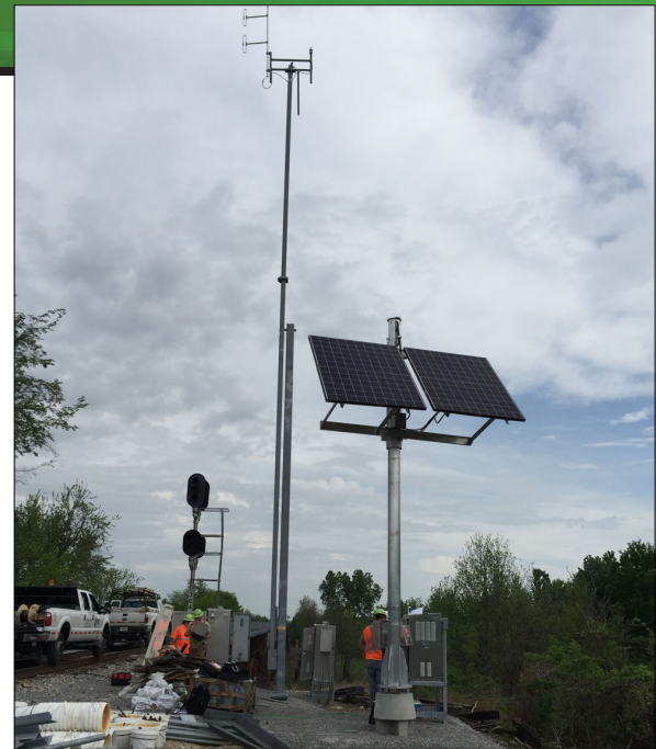
1060W Solar System w/RP Series Retractable Mast
